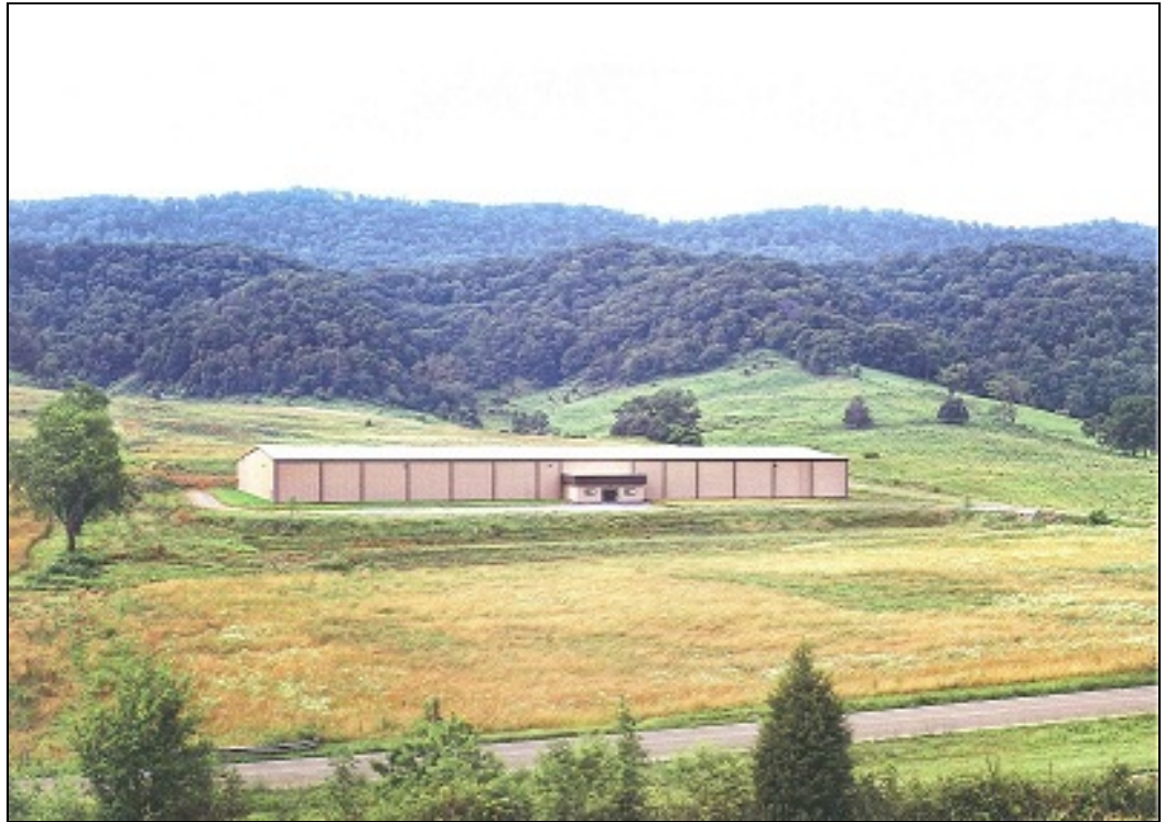
Constitutional Oaks Shell Building
