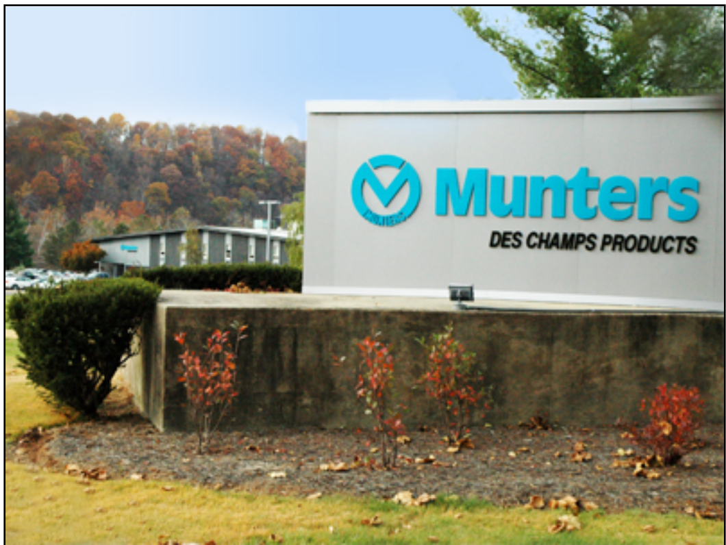
Munters Manufacturing Facility
